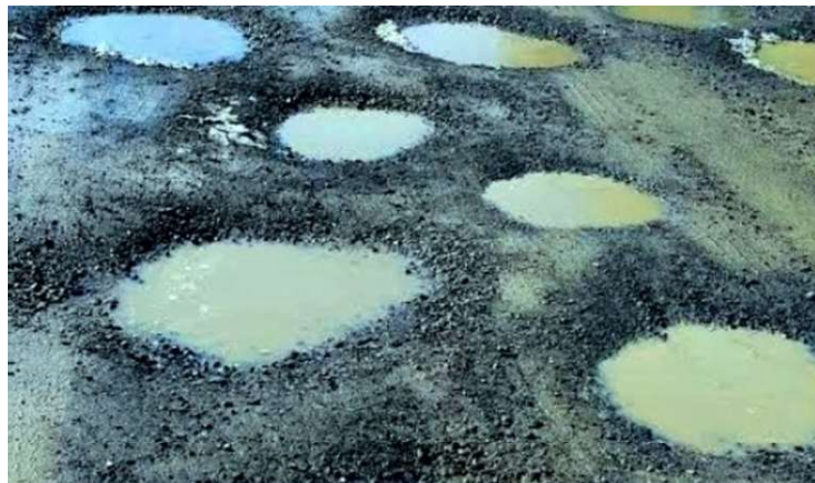
Figure 1. Road Pothole [3]
