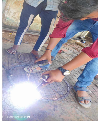
(ii) Welding Grate
