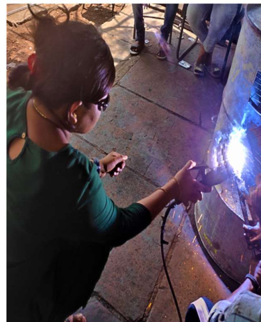
(iv) Welding Grate to Drum
