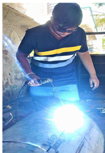
(v) Welding the Hinges and Door
